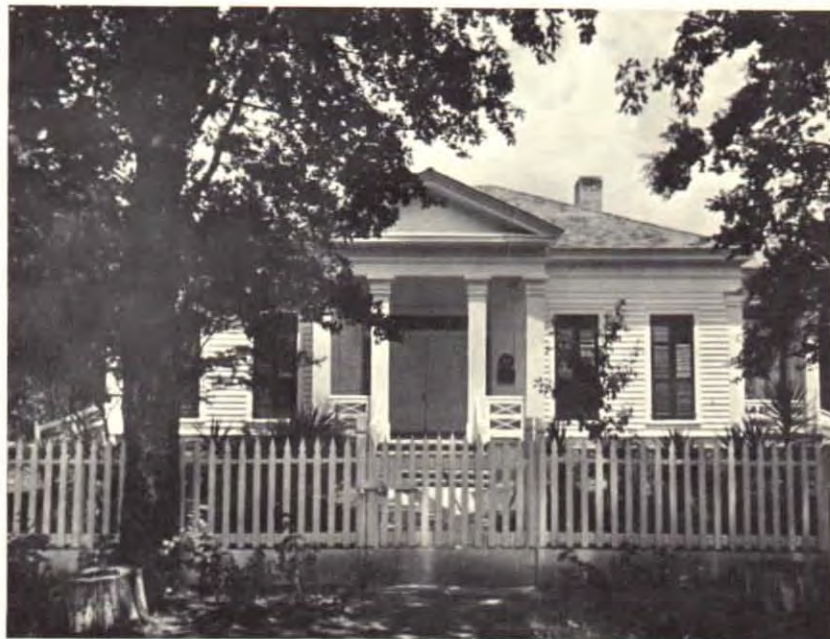
The Bradley House since restoration.
